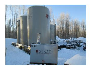
Glycol heaters are an environmentally friendly source of heating as their footprint can be as little as 1/8th the size of a traditional boiler building.
